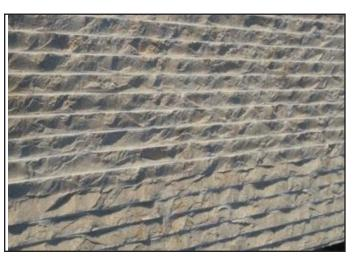
**Striped:** A Stone finish with parallel grooves cut into it. Available with 1-4 grooves to the inch (254mm), the finish may be executed by hand (hand-tooled) or machine (machine-tooled)
